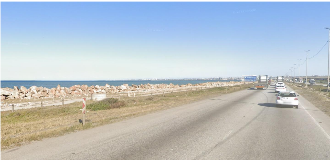
Figure 3: Google Earth street view of the site from the southbound N2 route.
